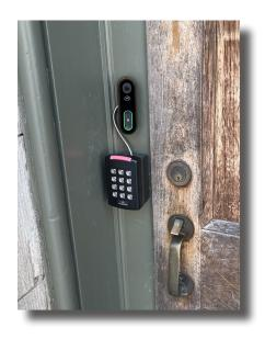
The Access Control system by I Touch AVS is in the process of being installed and configured on the front door of the Parish Hall. Please bear with us as we complete the installation process, WiFi upgrade, conduit reconfiguration, PIN distribution and training for using the system. You may continue to use physical keys until notified to return them.
